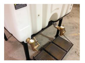
7. Install poly elbow(s) into stacked tank drain port(s). Angle poly elbows at a 5 o'clock position, aiming to its corresponding stand elbow kit. Repeat as necessary.
