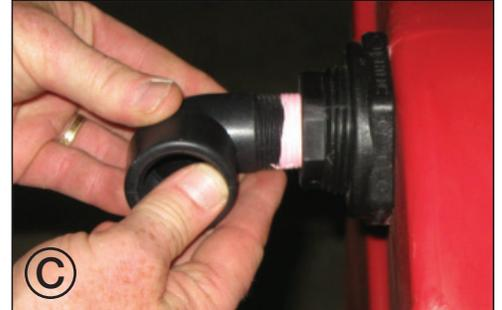
Attach the overflow elbow to the other end and hand tighten.
