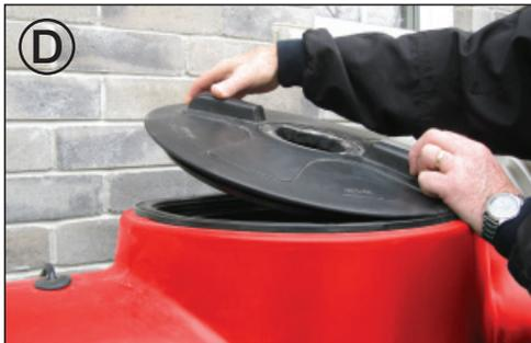
Place the access cover in place and lock into position.
