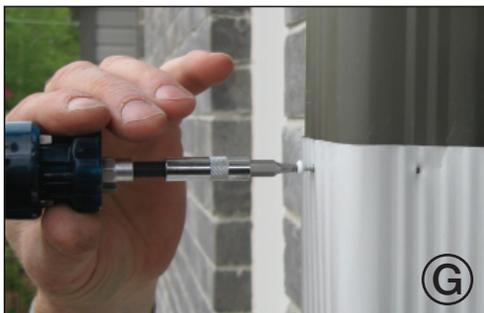
Using the provided screws attach the leaf catcher to the downspout. Use two screws at this connection.
