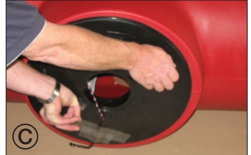
Unscrew the access cover. Note the arrow markings on the cover for proper rotation.
