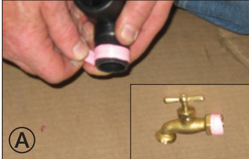
Using the provided roll of teflon tape wrap the threads of both the spigot and the overflow elbow.
