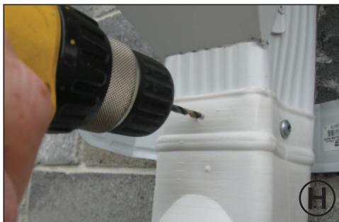
Place the flexible downspout in position, drill and attach it using the provided hardware. Use two screws at each this connection.
