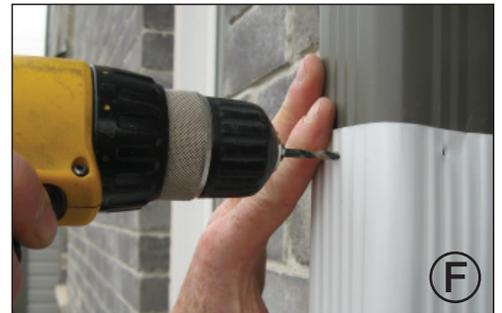
Cut the existing downspout to roughly 5-1/2 ft. from the ground. Place the leaf catcher in position. Using a 1/8" drill bit, drill through both.
